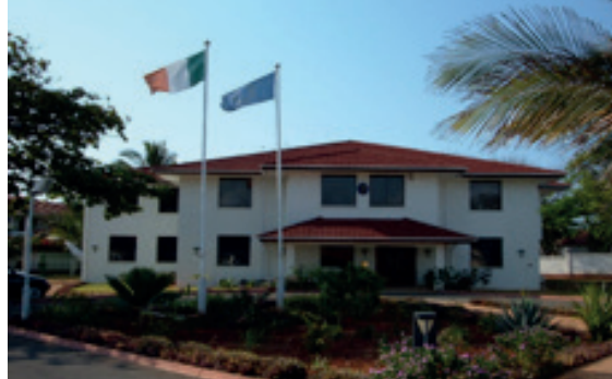
Embassy of Ireland, Dar es Salaam
